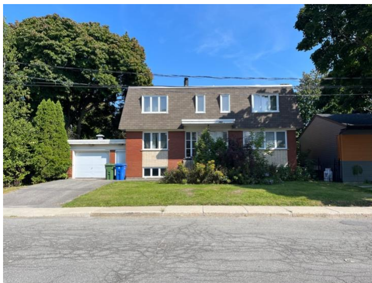
Front of the Rectory
