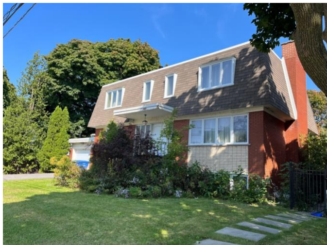
Front of the Rectory
