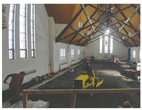
Church interior demolition (removing the old concrete floor in preparation for pouring a new concrete floor).
